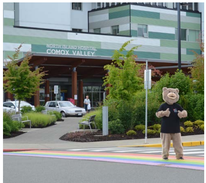
North Island Hospital - Comox Valley
