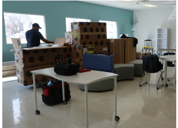
Fresh paint and new furniture being delivered for the Youth Centre
